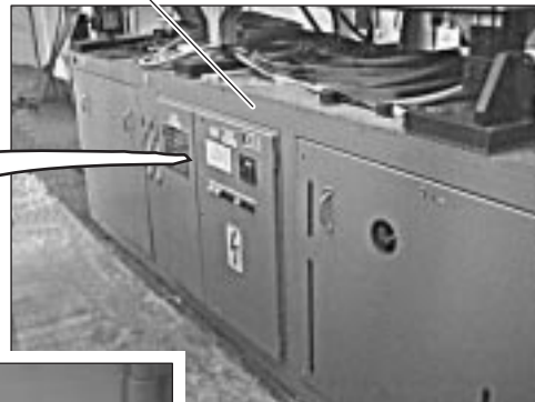
Verify Chiller Operator's Panel Turns On
