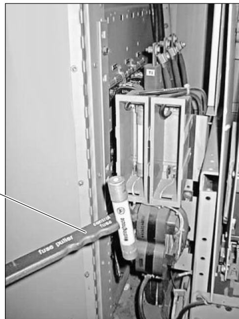
Removing a Primary Side Control Circuit Fuse
