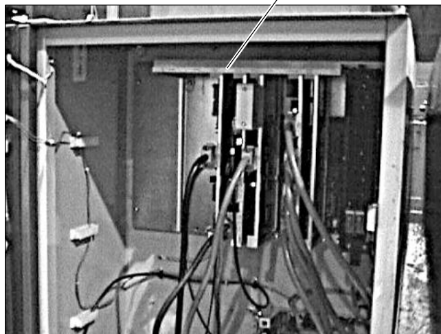
Example of Retaining Device
