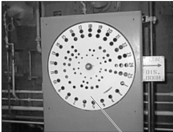
Photoelectric Switch is Behind Wheel
