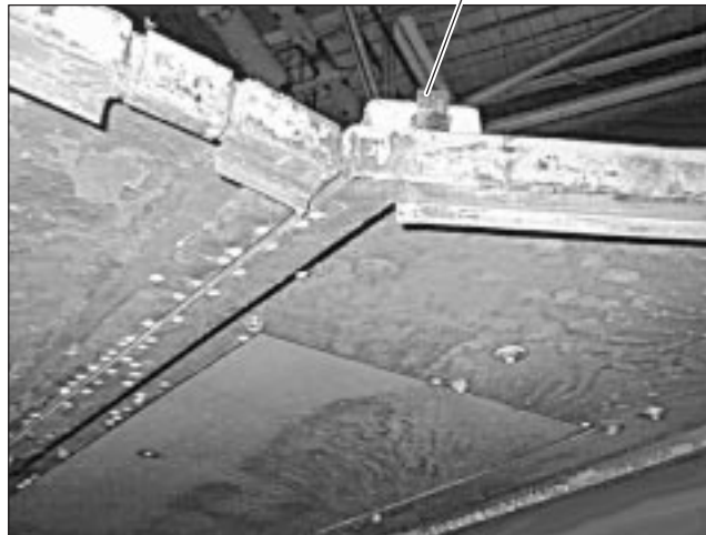
Blocked Proximity Switch (Top of Machine)
