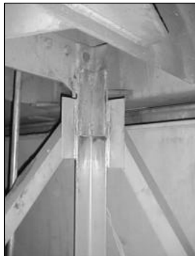
Check Braces for Cracks
