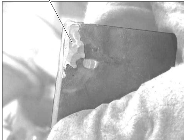
Brazed Surface After Grinding
