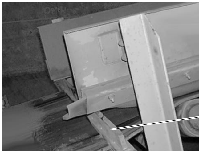
Belt Clamp in Place to Block Belt Movement
