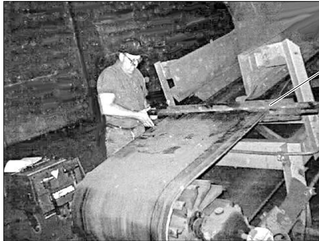
Belt Clamp Being Installed
