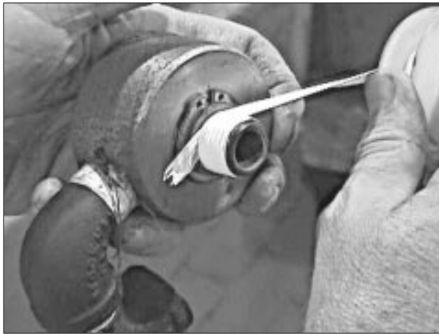
Proper Tape Application
